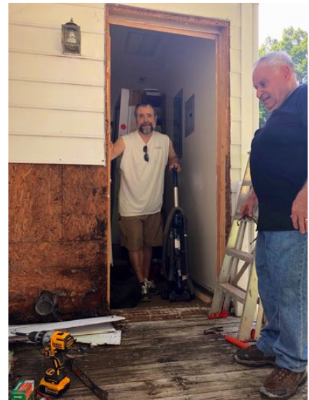
Ripping out rotten wood
